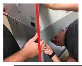
Be sure to line up the sides and the rear of the machine as flush as possible to align at least 4 screws with their pre-threaded holes.
